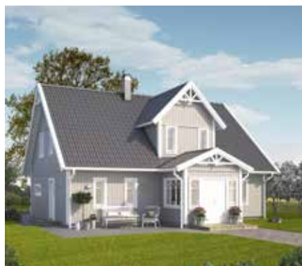
The classic entrance vestibule is coming back into favour and is now serving as a "heat sluice".
