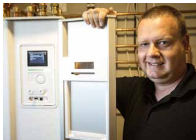
"Electricity will not get cheaper in the future, so I wanted to take this opportunity to invest in the sun's free heat while we were building", says Joakim Wulf in Hjärnarp. Joakim heats 270 sqm using a NIBE F2026 air/water heat pump, 3 x 24 pipe IntelliHeat solar panels and a NIBE VVM 500 Indoor unit.
