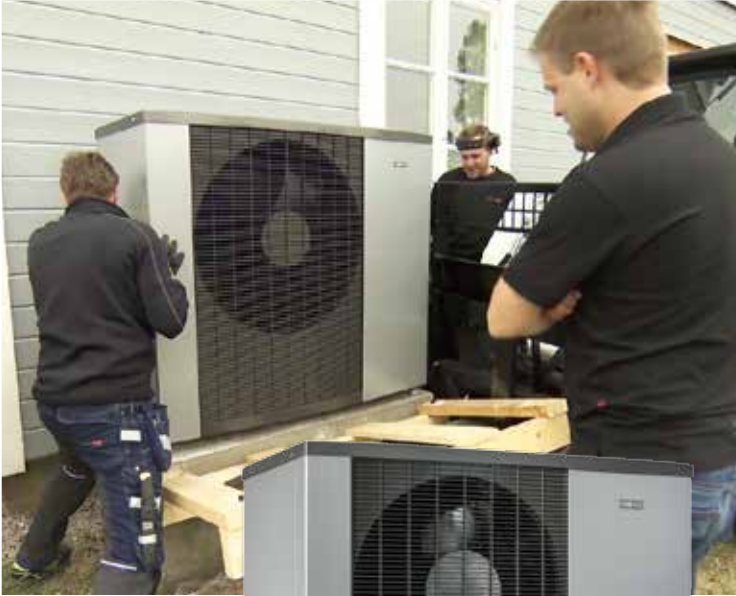
A new NIBE F2120 being installed.
